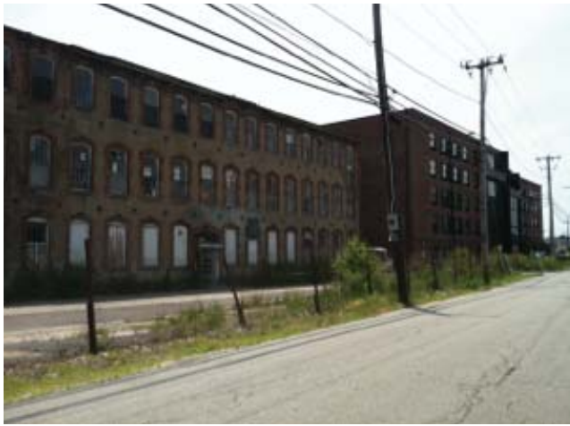
The vacant Pontiac Mills structure has the potential for reuse, and sits next door to the new NYLO Hotel.
